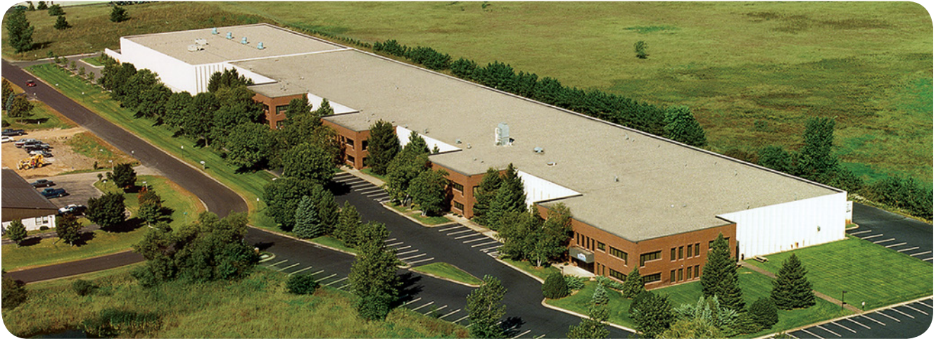
Cat Pumps occupies 149,000 sq. ft. at its world headquarters in Minneapolis, MN.
